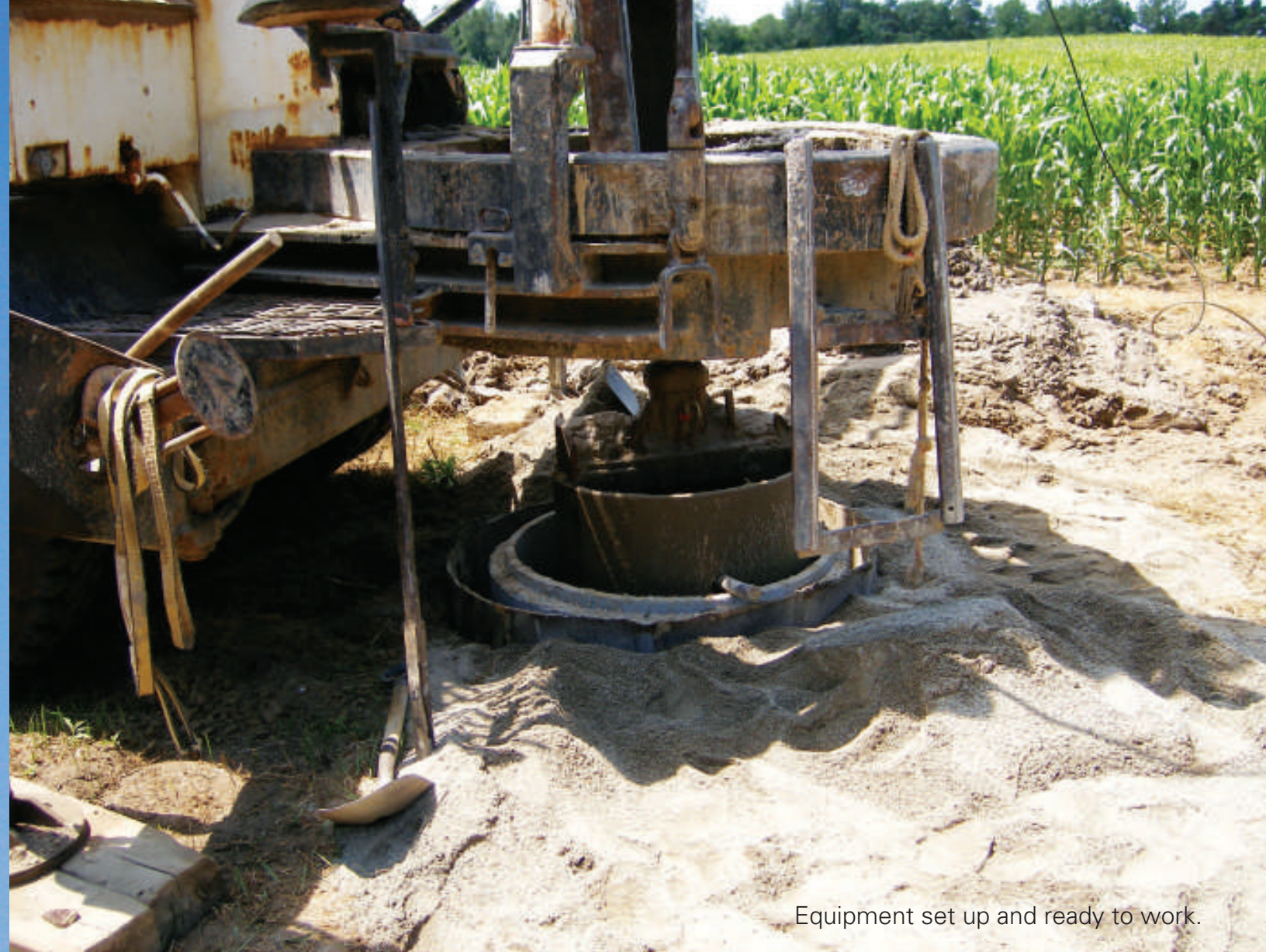
Mast set up. Despite how it looks, the proper set back from overhead wires was maintained.
